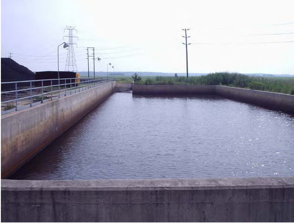
Concrete Detention Basin for Coal Pile
