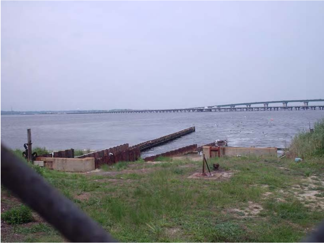
Intake from River
