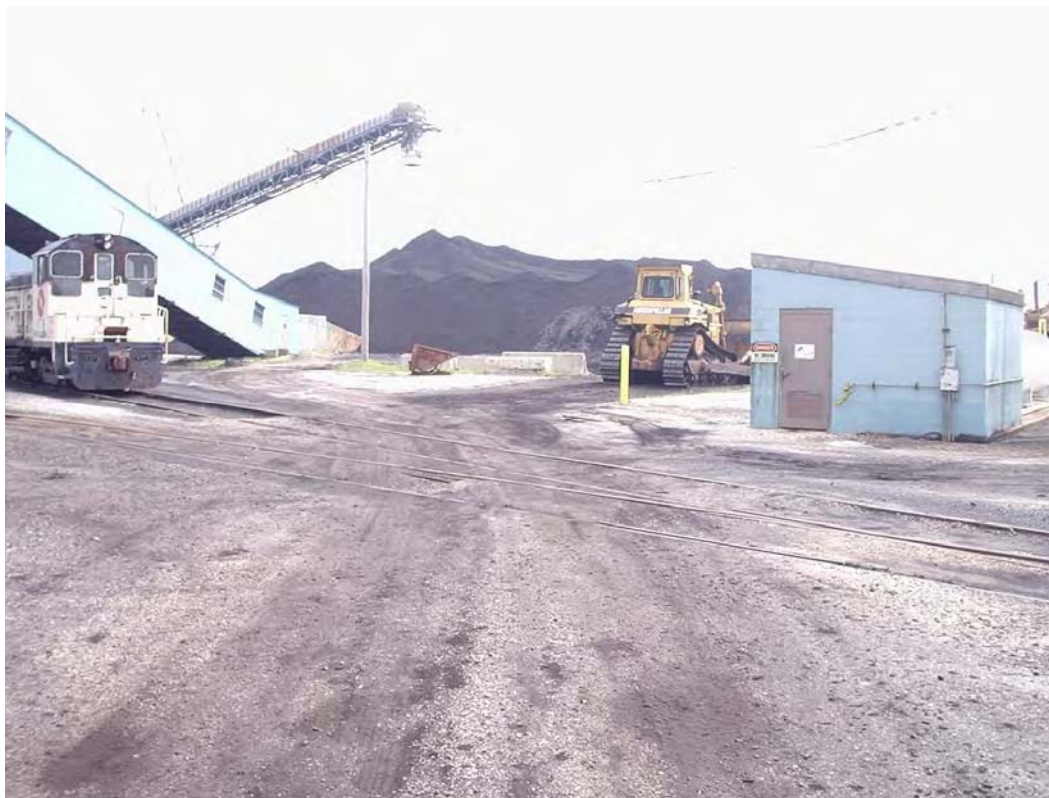
Coal Storage Pile
